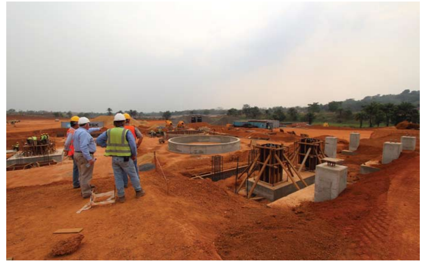
Above Construction of Marampa processing plant
